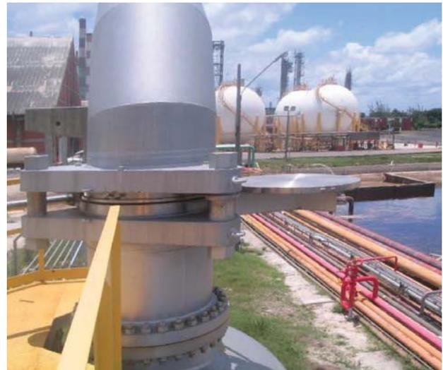
Cam-Set® DN 500 (20"), ASME 150# with spectacle plate support
